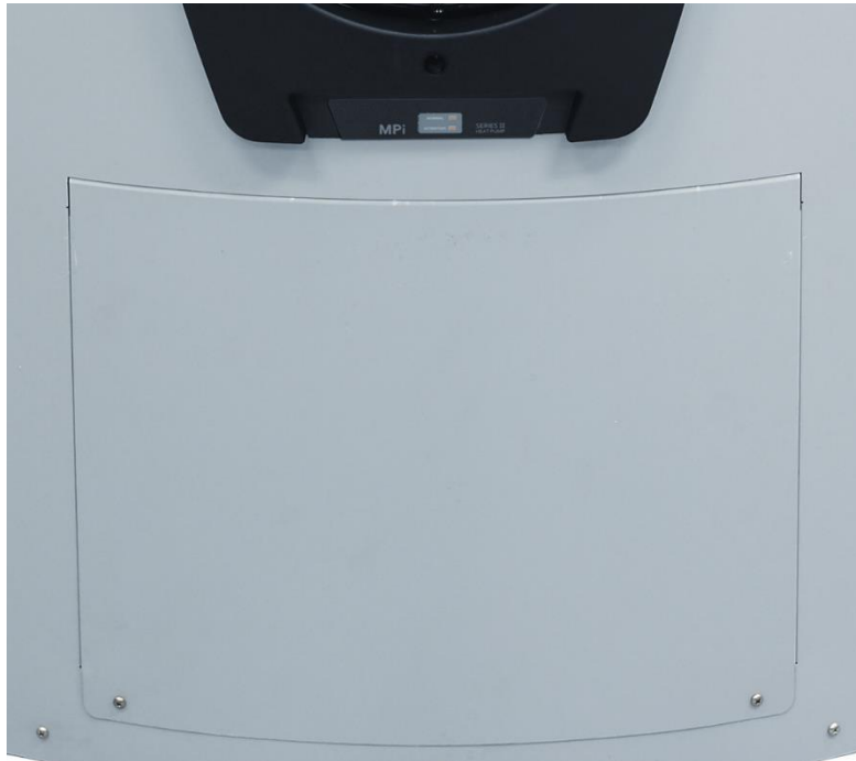
Step 27 replace heat pump module front cover
