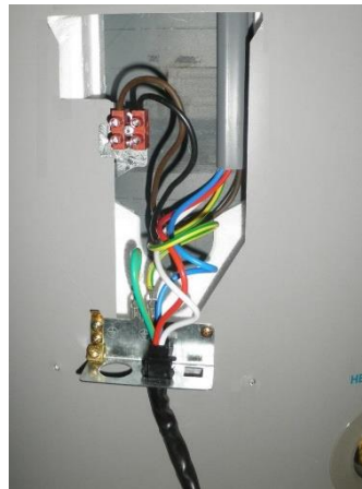
Step 3 withdraw the power cable
