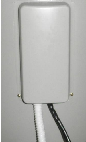
Step 5 refit lower front cover
